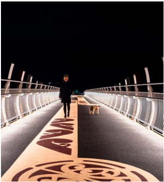
He Ara Kotahi Bridge
